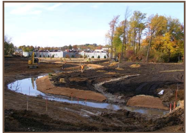
Stream Restoration in the South Zone
