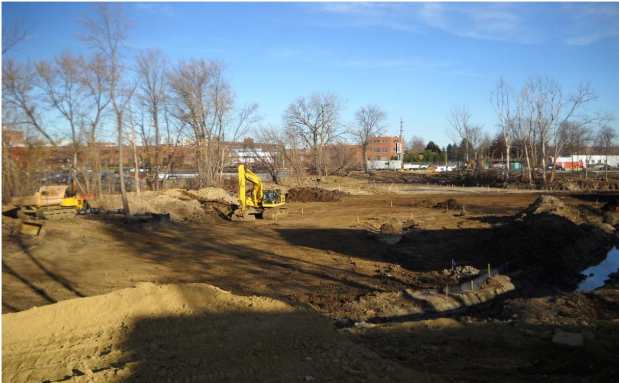
Photo #32: North Zone undergoing restoration
