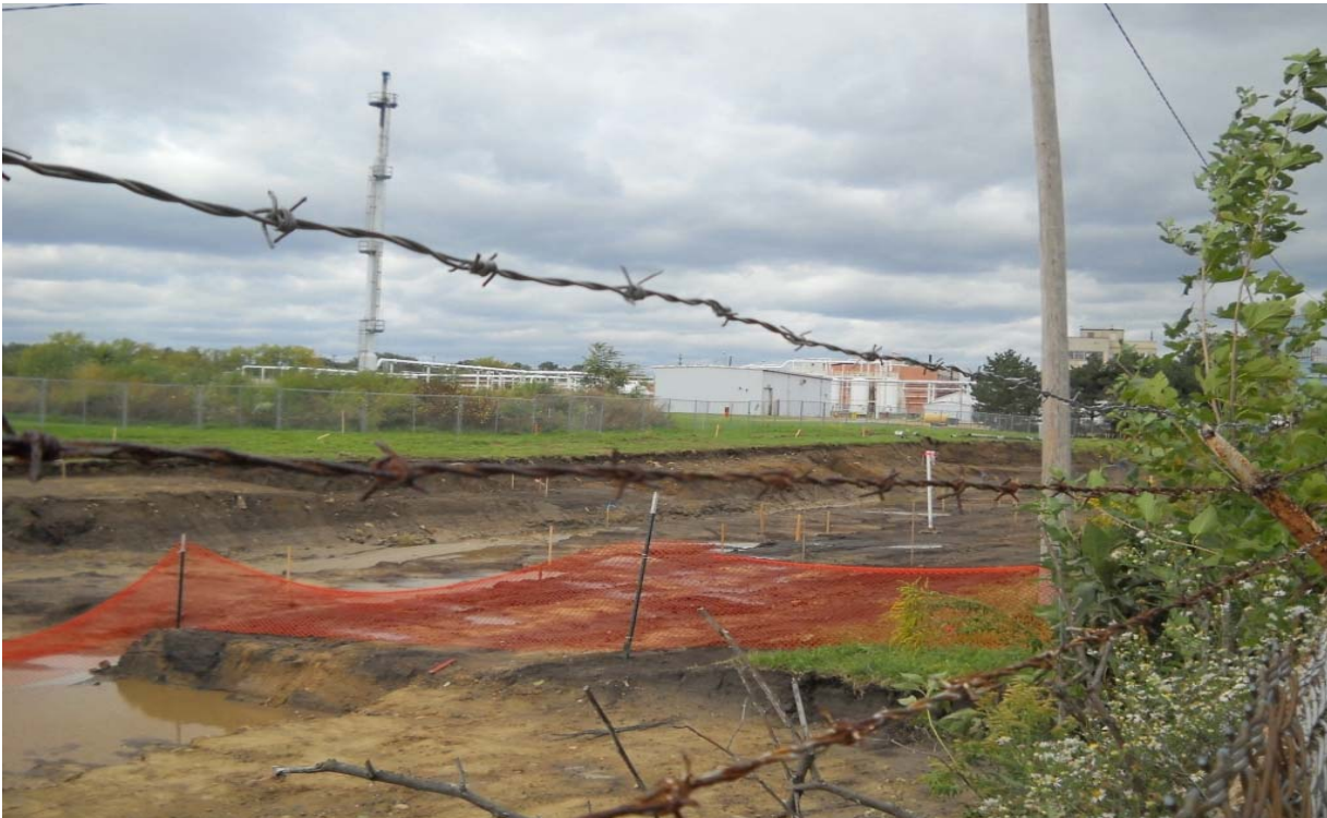
Photo #26: Middle Zone excavation with verification sample locations staked
