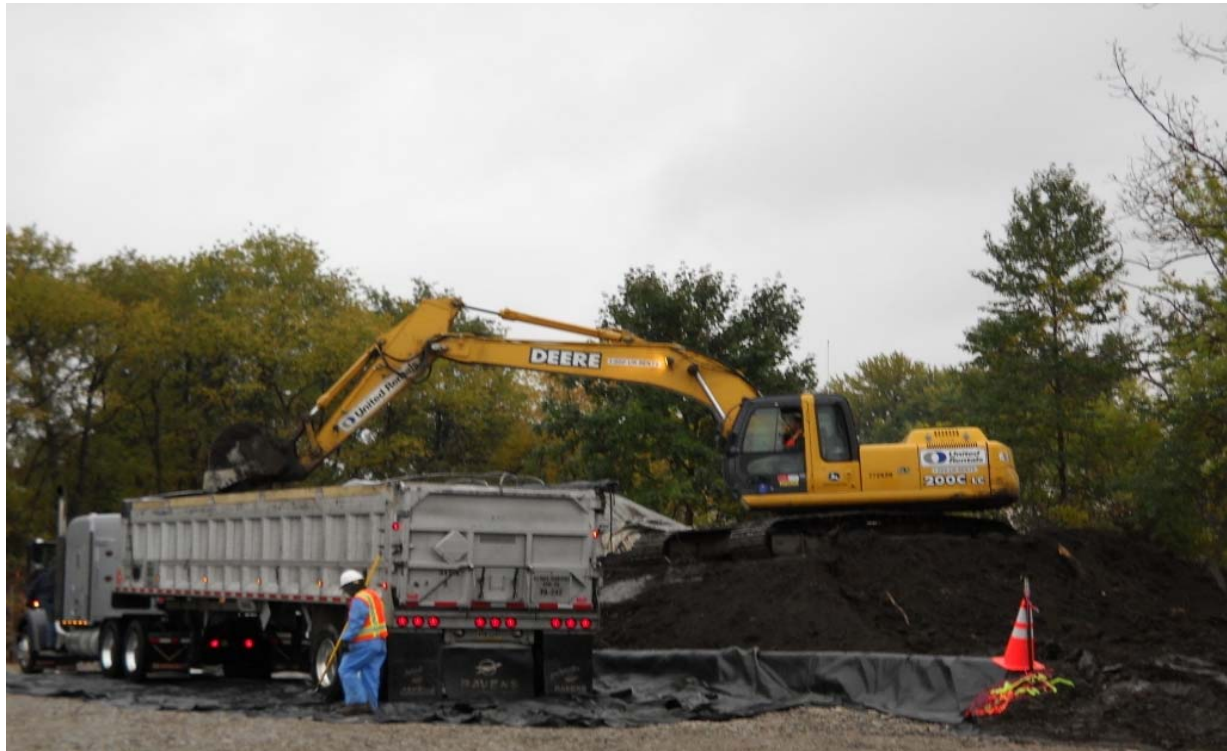
Photo #29: North Staging Area truck loading operations
