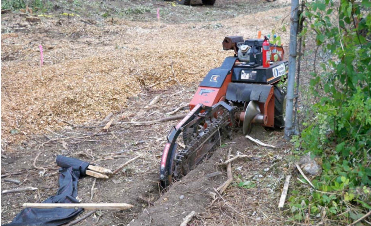
Photo #11: Installation of silt fence prior to excavation activities
