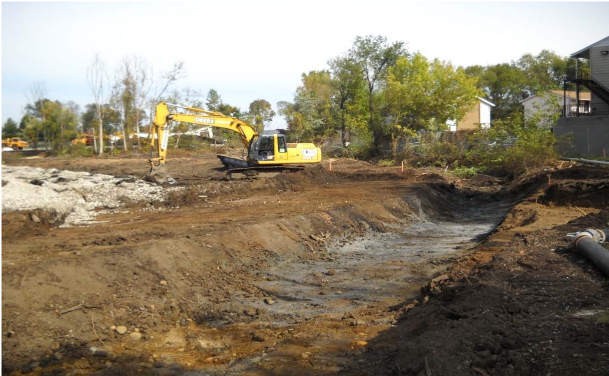
Photo #28: North Zone channel excavation
