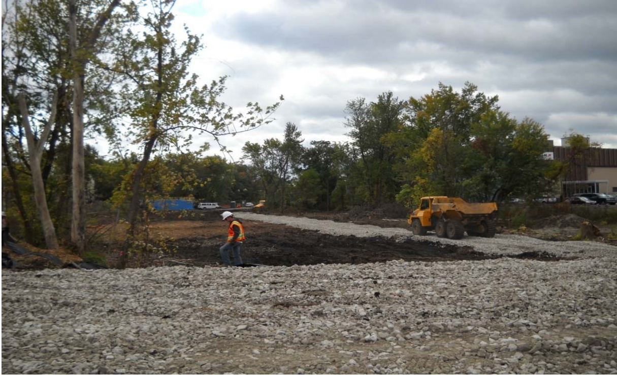
Photo #15: North Staging Area and temporary stone access road
