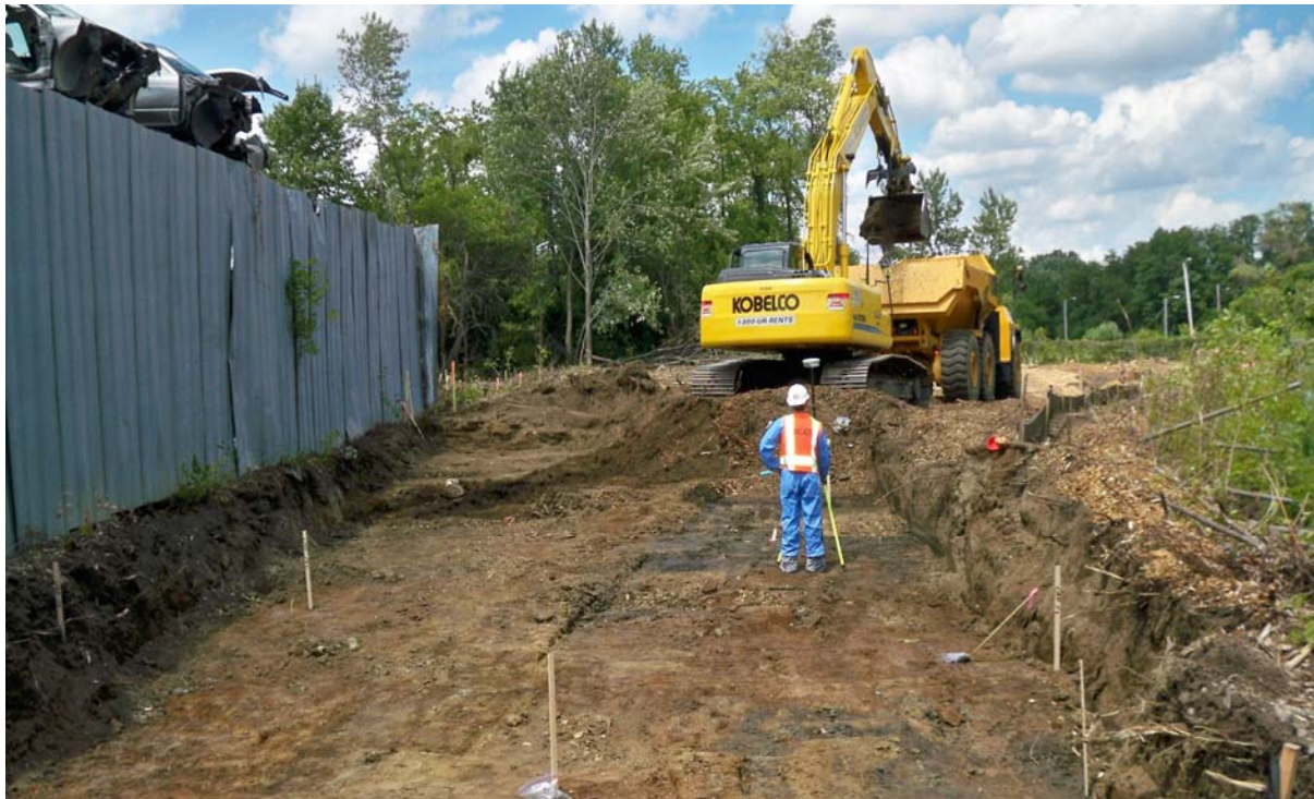
Photo #20: South Zone soil excavation and loading
