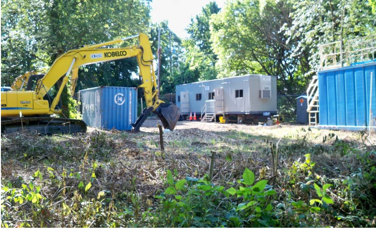
Photo #5: South Staging Area
