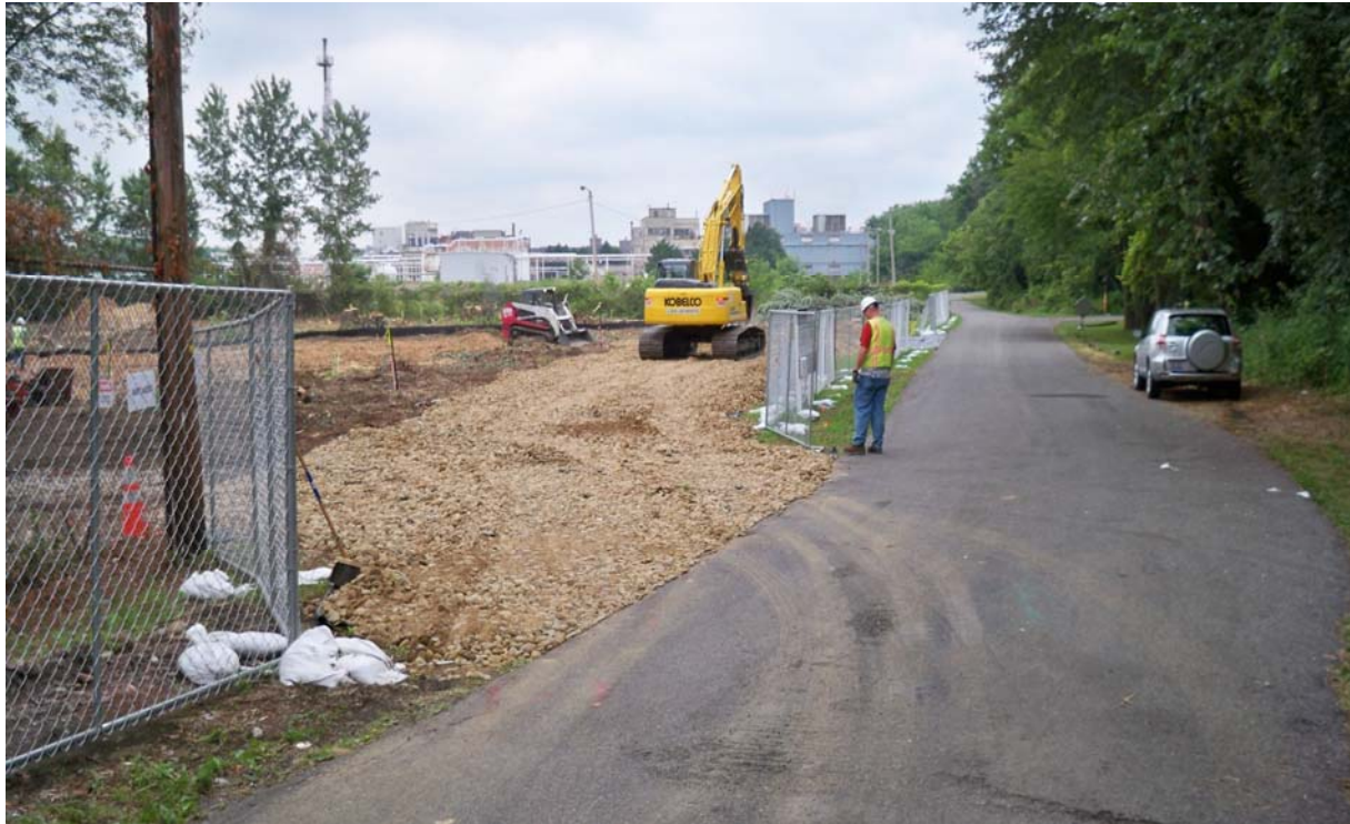
Photo #9: South Zone construction entrance
