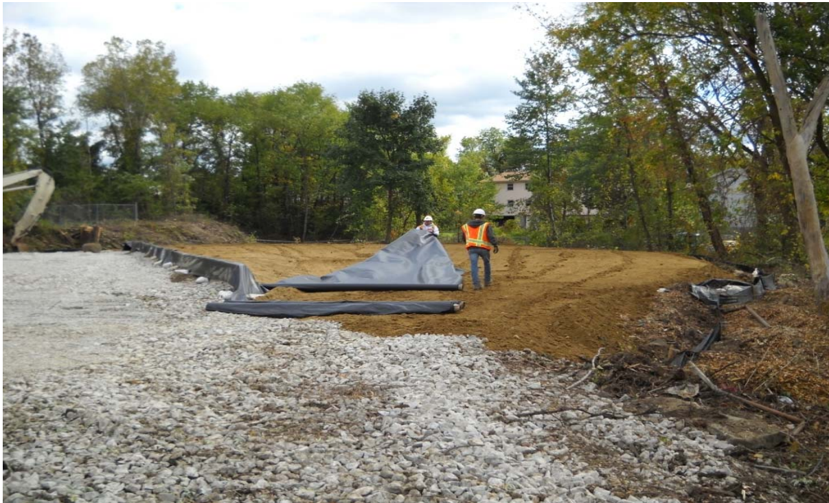
Photo #6: North Staging Area and lined soil stockpile construction
