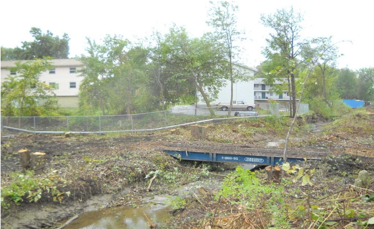
Photo #14: Temporary bridge used for stream crossing
