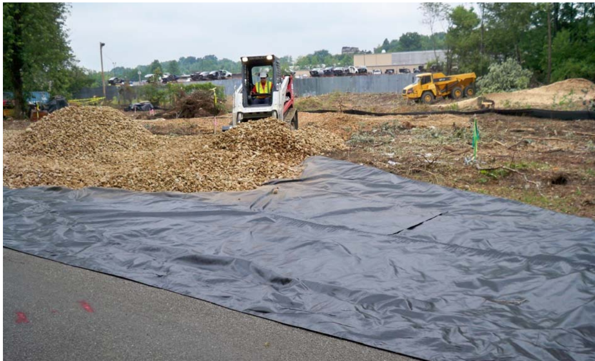
Photo #8: Construction of lined truck loading area in the South Zone
