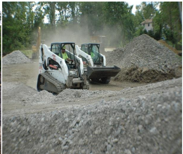
Materials for the restoration are stockpiled
