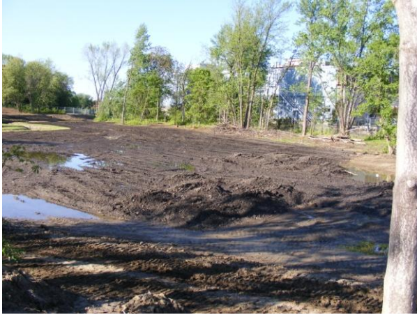
Top soil work in wetland area – early May
