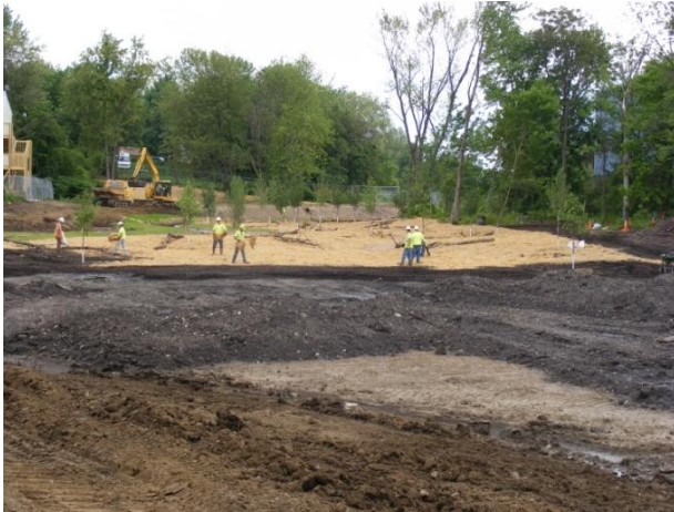
Subgrade work on eastern edge of project
