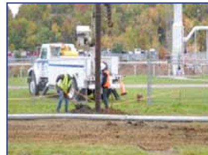
Workers set one of the light poles on IRG property.
