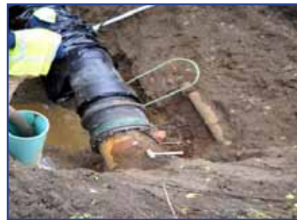
The relocation of the 20 inch water main.
