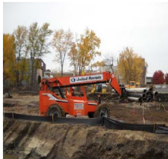
5. Removing pump bypass piping from the northern portion of the site.
