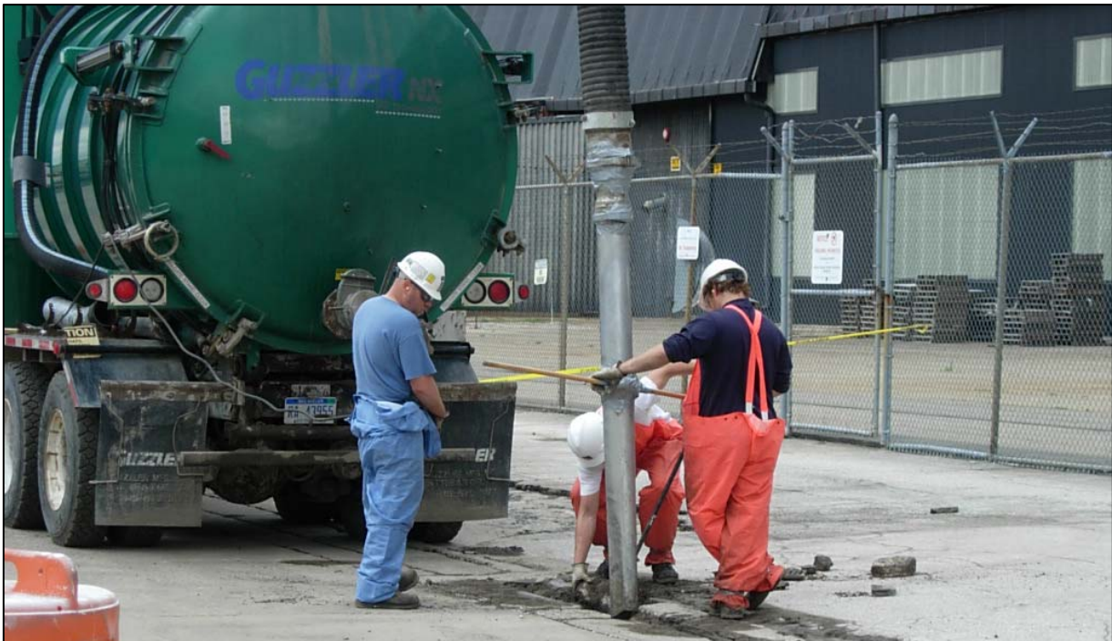
Photo 3 – Hand lance vacuum process removal
