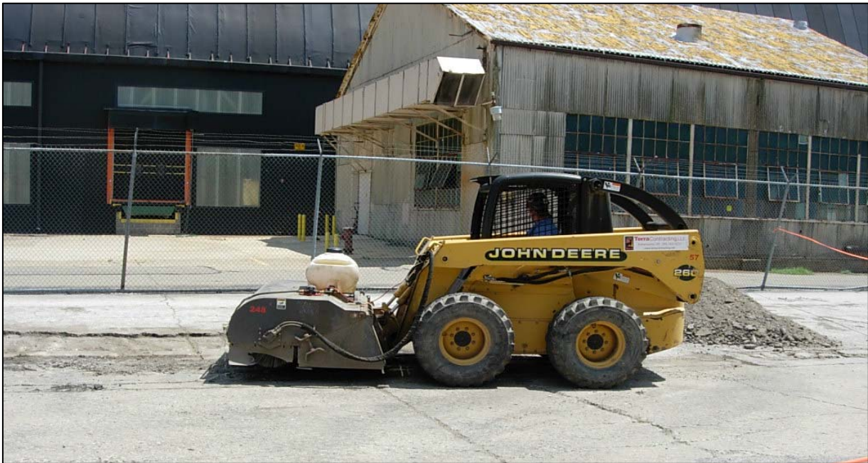
Photo 2 - Skid Steer debris removal operation
