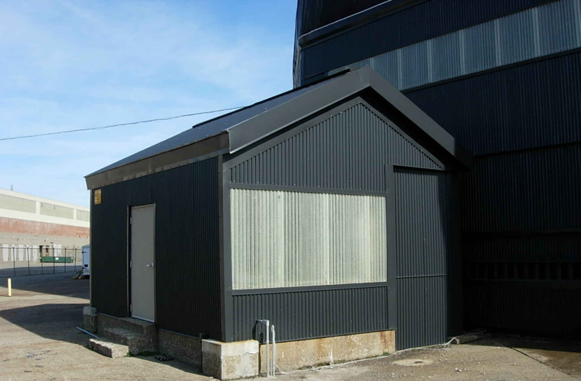
South West Motor House, October 2006
