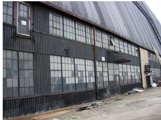
Typical Airdock vertical siding
