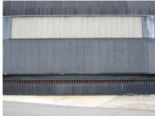
Typical Airdock door siding
