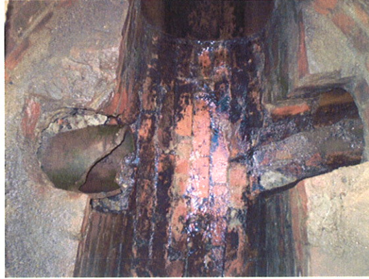
Manhole PAE-1 After Debris Removal
