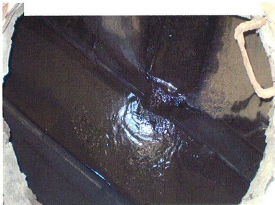
Manhole MH-1 Before Debris Removal
