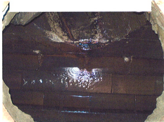
Manhole MH-1 After Debris Removal
