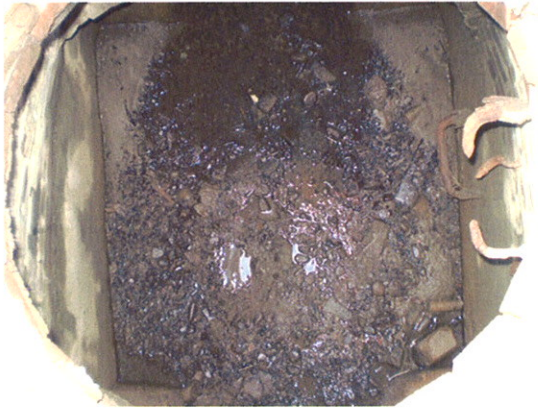
Manhole PAW-48-5 Before Debris Removal
