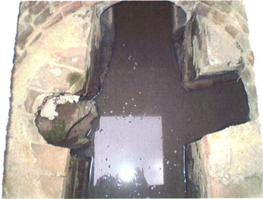
Manhole PAE-1 Before Debris Removal
