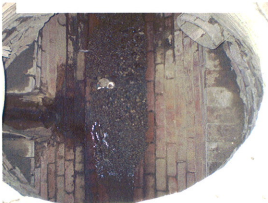
Manhole PAW-6 Before Debris Removal
