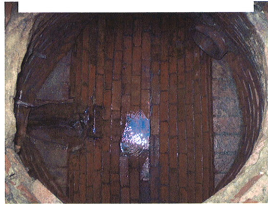
Manhole PAW-6 After Debris Removal
