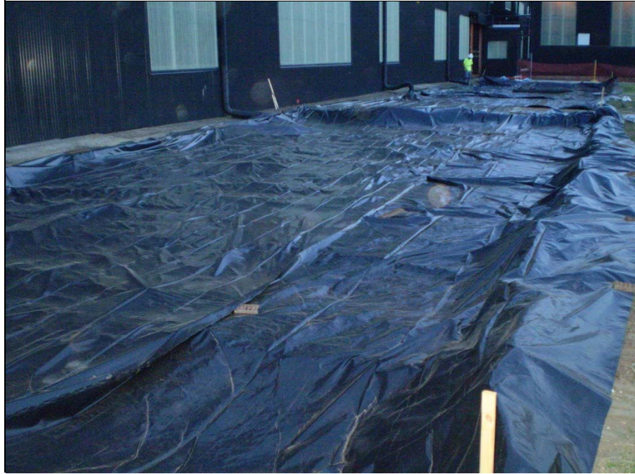
Photo # 3: Facing north, excavation covered awaiting sample results.
