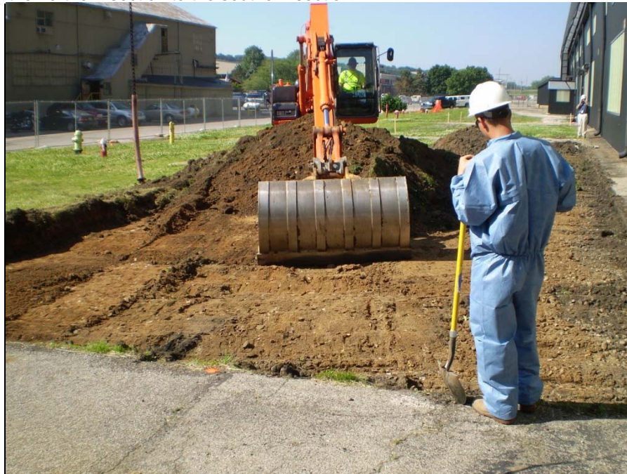
Photo # 2: Facing south-Continuation of excavation activities in the Southeast Area.
