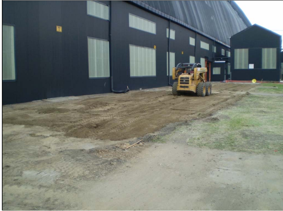
Photo # 5: Backfill in the Southeast area is being spread and compacted.
