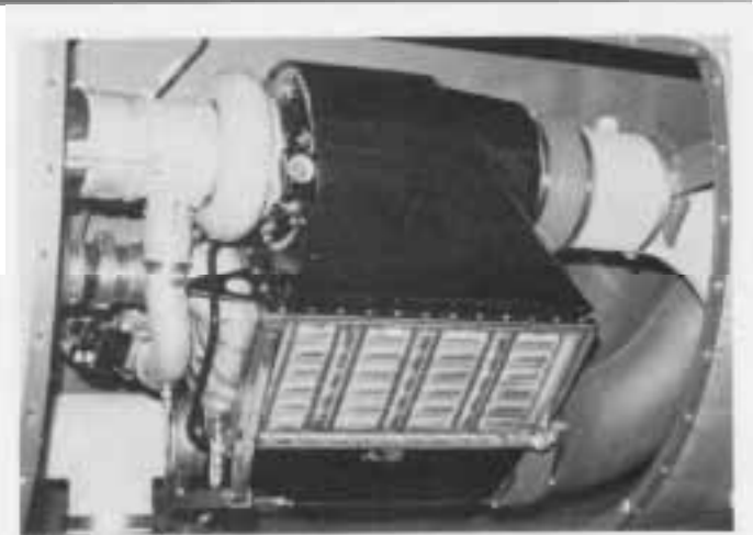
Cargo compartment air conditioning unit forward right wheel well fairing.
