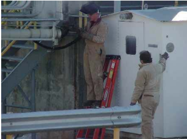
Use of Step Ladder as Straight Ladder
