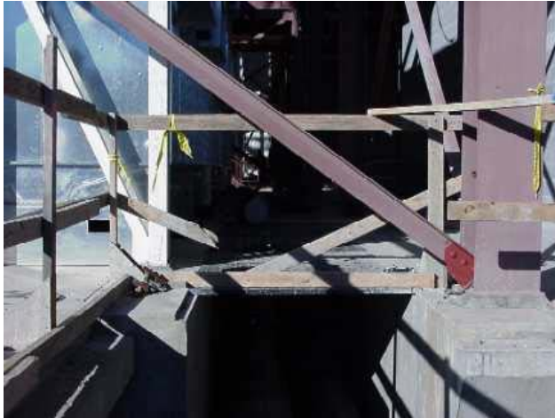
Non-Compliant Guardrail
