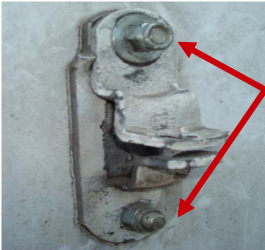
Different Bolts / Loosen Hasp
