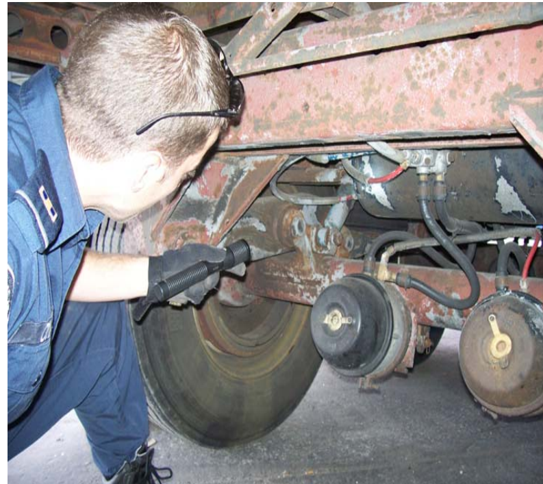
Trailer / Weld Marks
