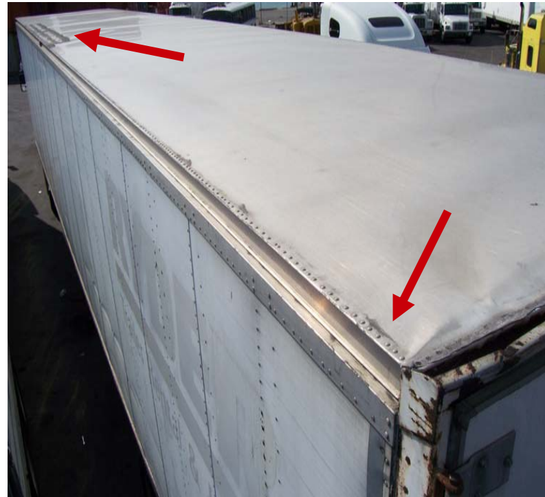
New Rivets / Repairs
