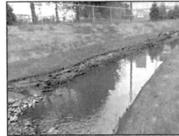
Figure 24. Brush Layering
